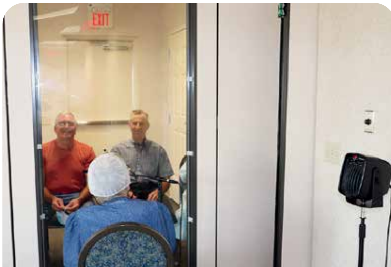
Residents and their families can visit safely in the conference room outfitted with a plexiglass barrier, a special sound system, and a separate ventilation system.
